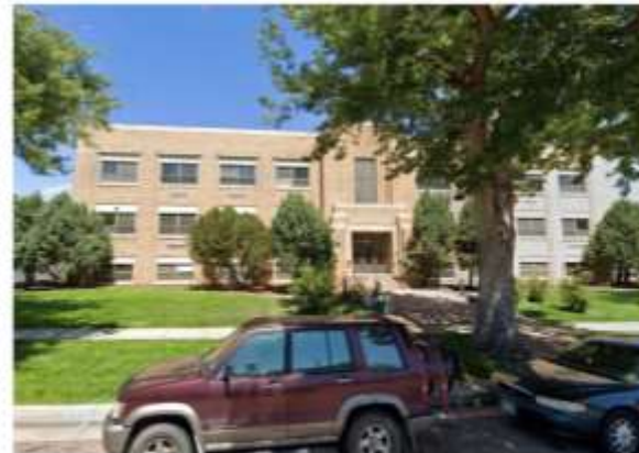
Apartment | Stoop, Entry Court
