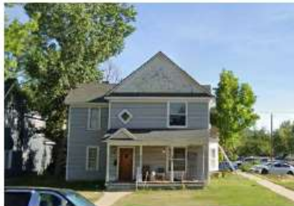
Porch | Full | Shed roof with gabel ornamentation
